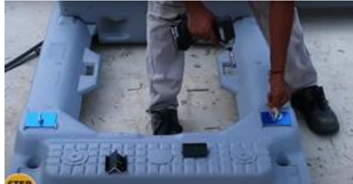
② Put the metal parts on the floats
