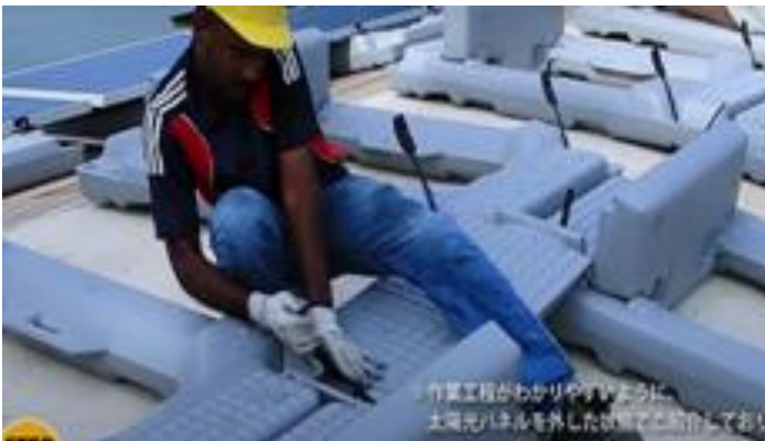
④ Connect the floats and the bridge with belts
