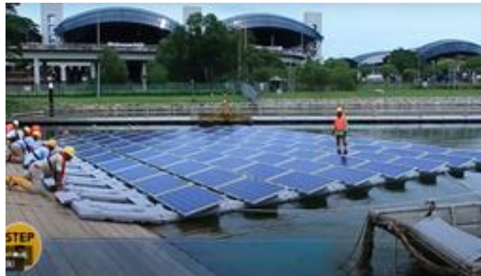
⑤ Put the floating solar panels on water
